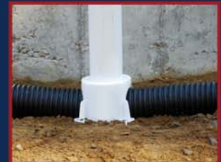
New Construction Installation
